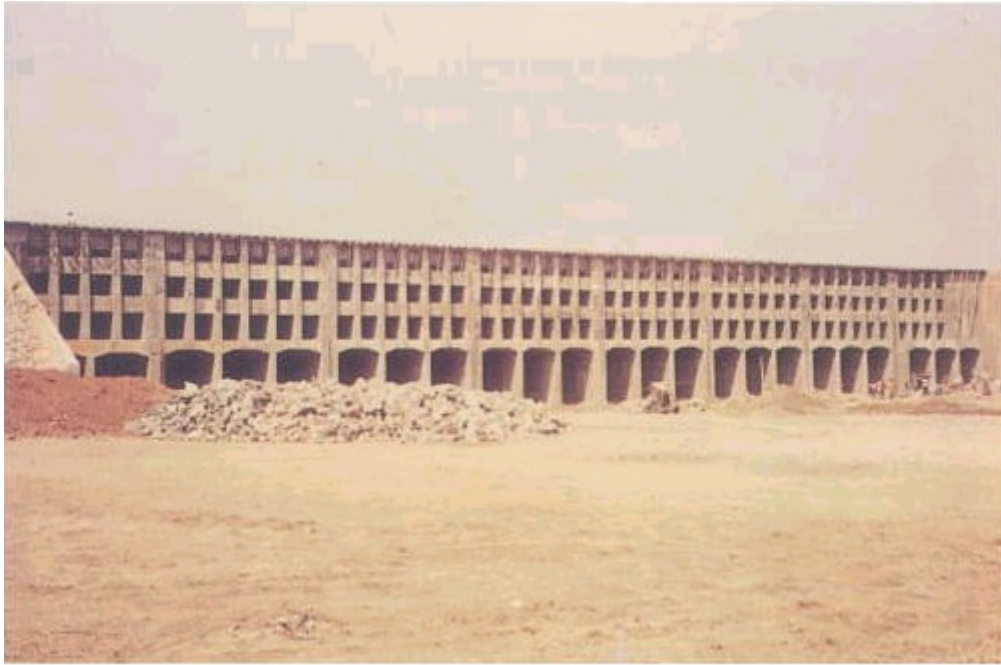
VIEW OF BOX TYPE AQUADUCT OF N.R.B.C FOR ALMETTY PROJECT (KARNATAKA)
