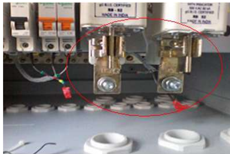
SMPS connections not provided
